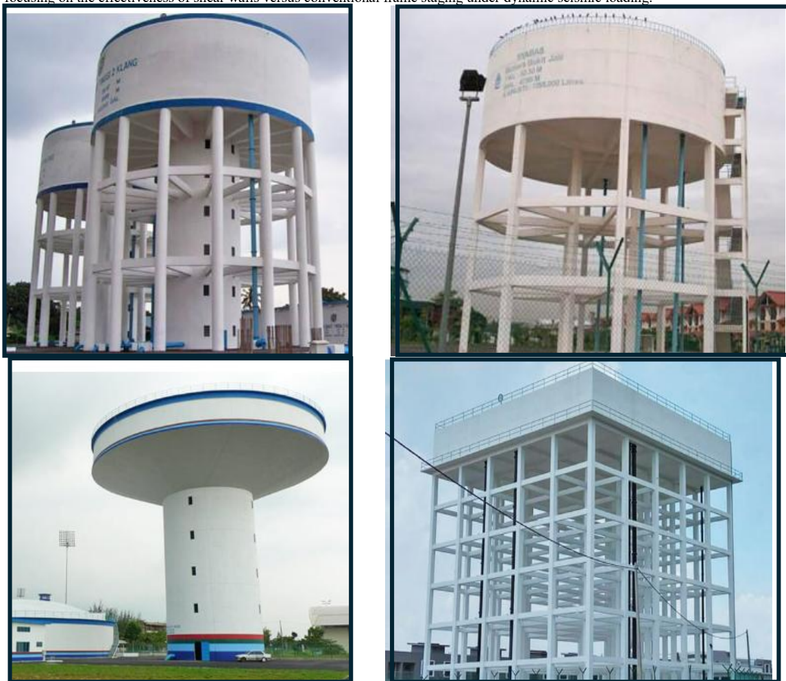
Fig.1.1: Elevated Water Tanks showing different staging configurations and shapes.
