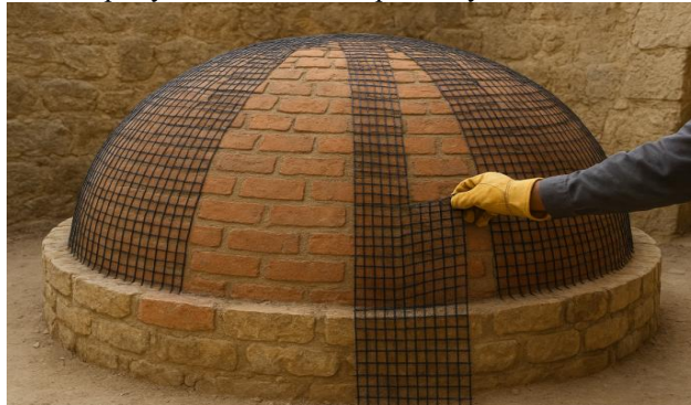
Fig5. Placement of textile mesh strips along dome surface.
