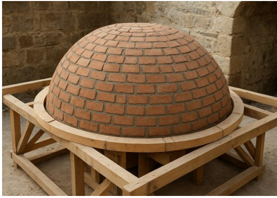
Fig3. Dome construction sequence (bricks laid over centering).
